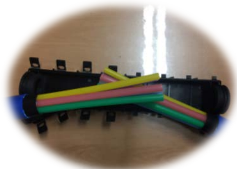
Complete sheath cutting on both microducts.
