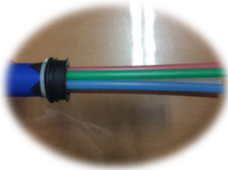
Insert microduct inside rubber cap and fix with cable ties.
