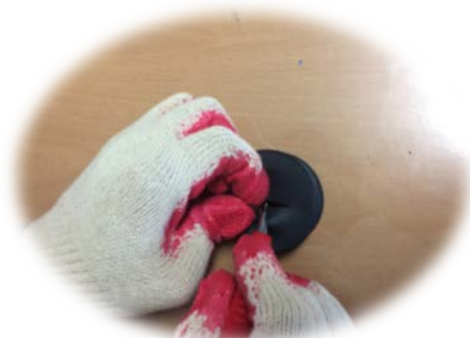
Make a hole of rubber sealing cap to fix the microduct.
