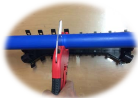
Cut the certain length of microduct to fix the closure size
