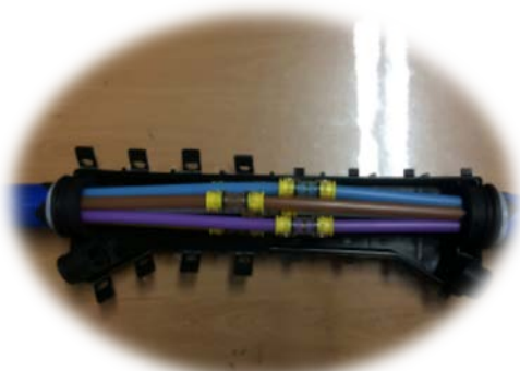
After microtubes connection, sort tubes in zip zap shape.
