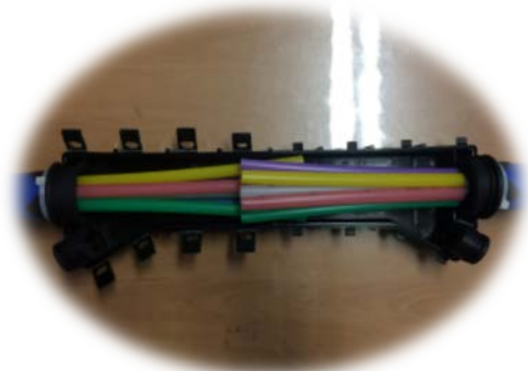
Align microtubes from both sides.
